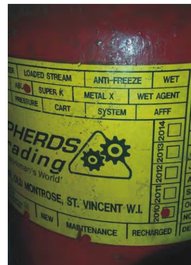
Non serviced fire extinguisher (last service date 6 years prior to date of inspection (2016))
