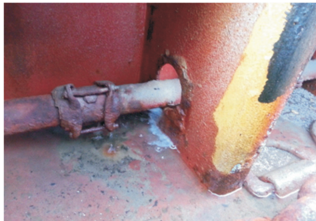
Main Fire Line Leaking
