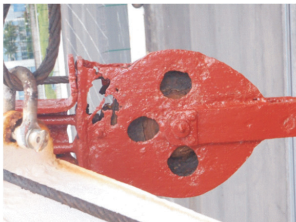
Life Boat Pulley Corroded
