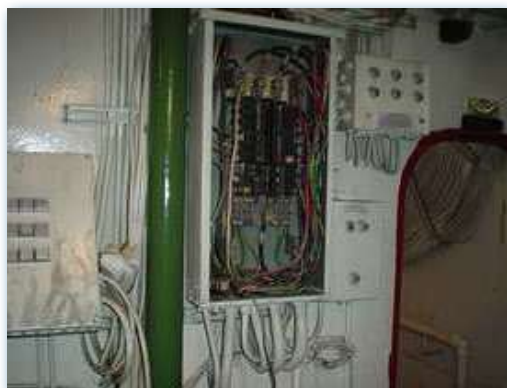
Exposed panel in engine room
