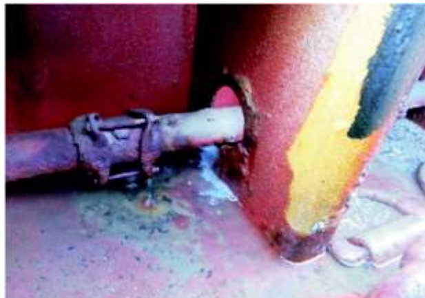
Main Fire Line Leaking
