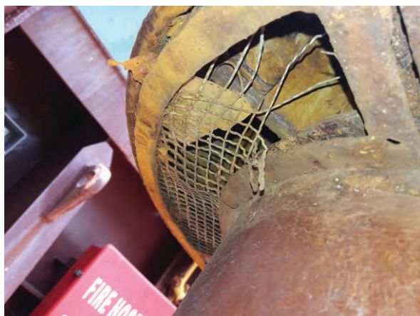
Damaged fire retardant screen for ventilator
