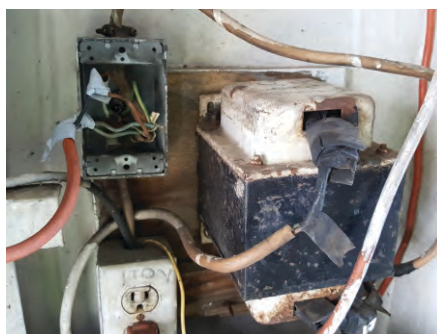
loose electrical wiring faults
