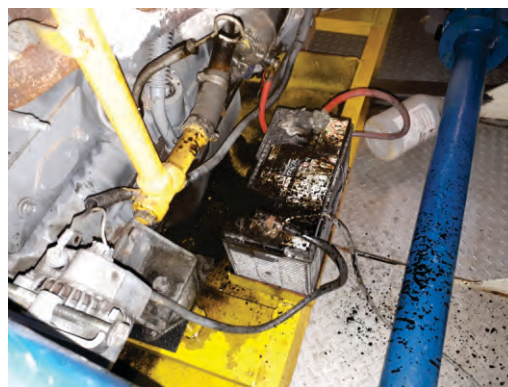
Oil leaking onto battery fire hazard
