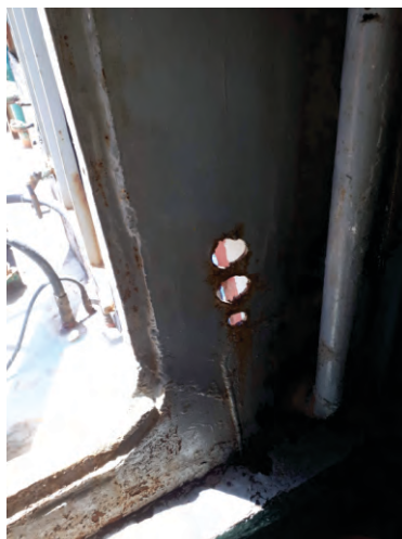
Bulkhead not weathertight
